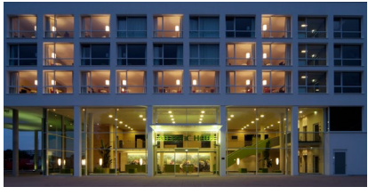
> ATLANTIC Hotel Galopprennbahn, Bremen
