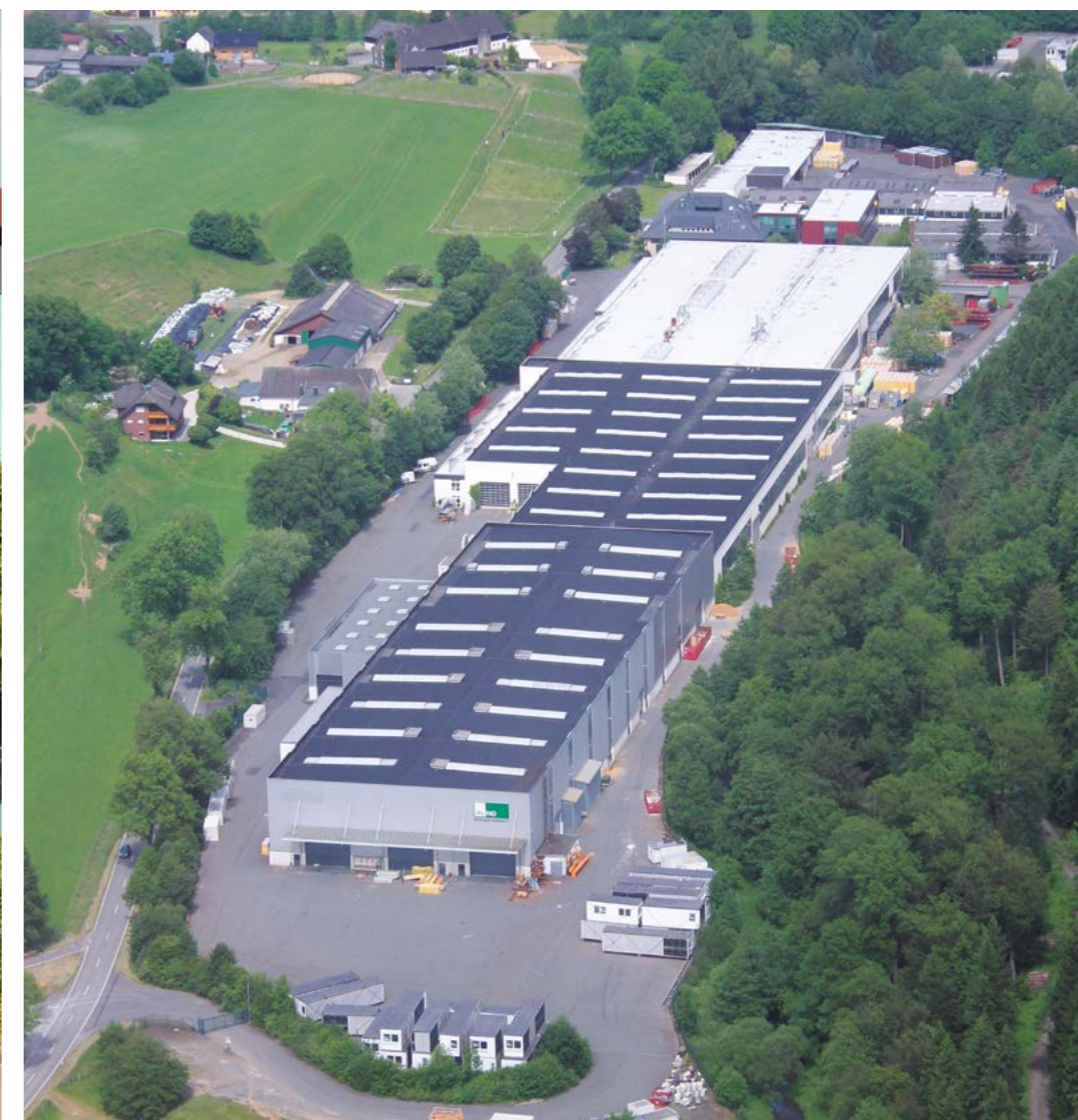
ALHO administration building and production unit at the Morsbach site
